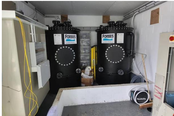
The two hydrogen peroxide storage tanks at the Nent Hags mine water treatment site.
